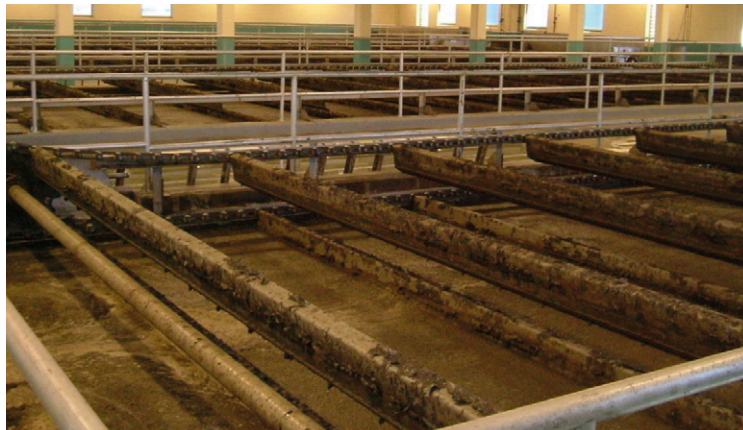
Fig. 7: Municipal waste water treatment plant Ohio, USA
