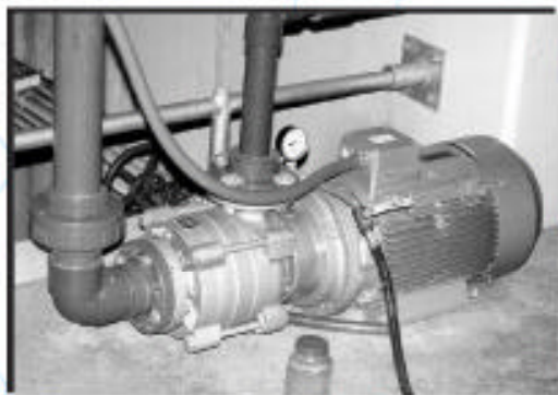
Installation of 30 HP EDUR DAF pump
